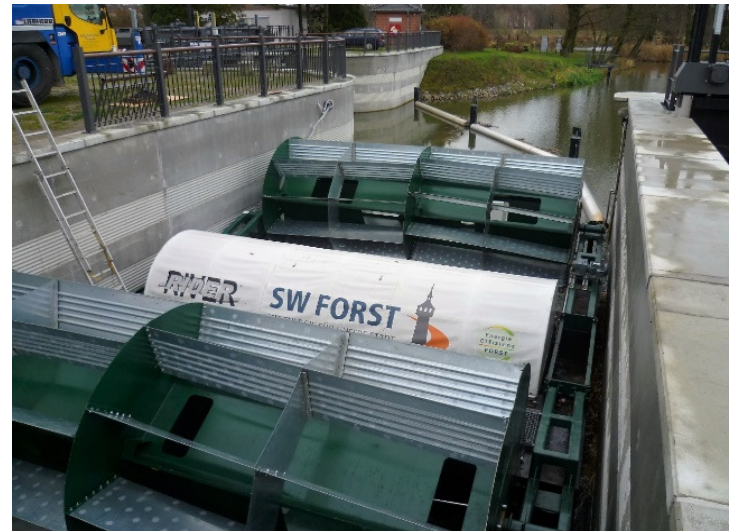
Figure 5 River Rider Tandem I (Forst/ Neiße) with technical specification
